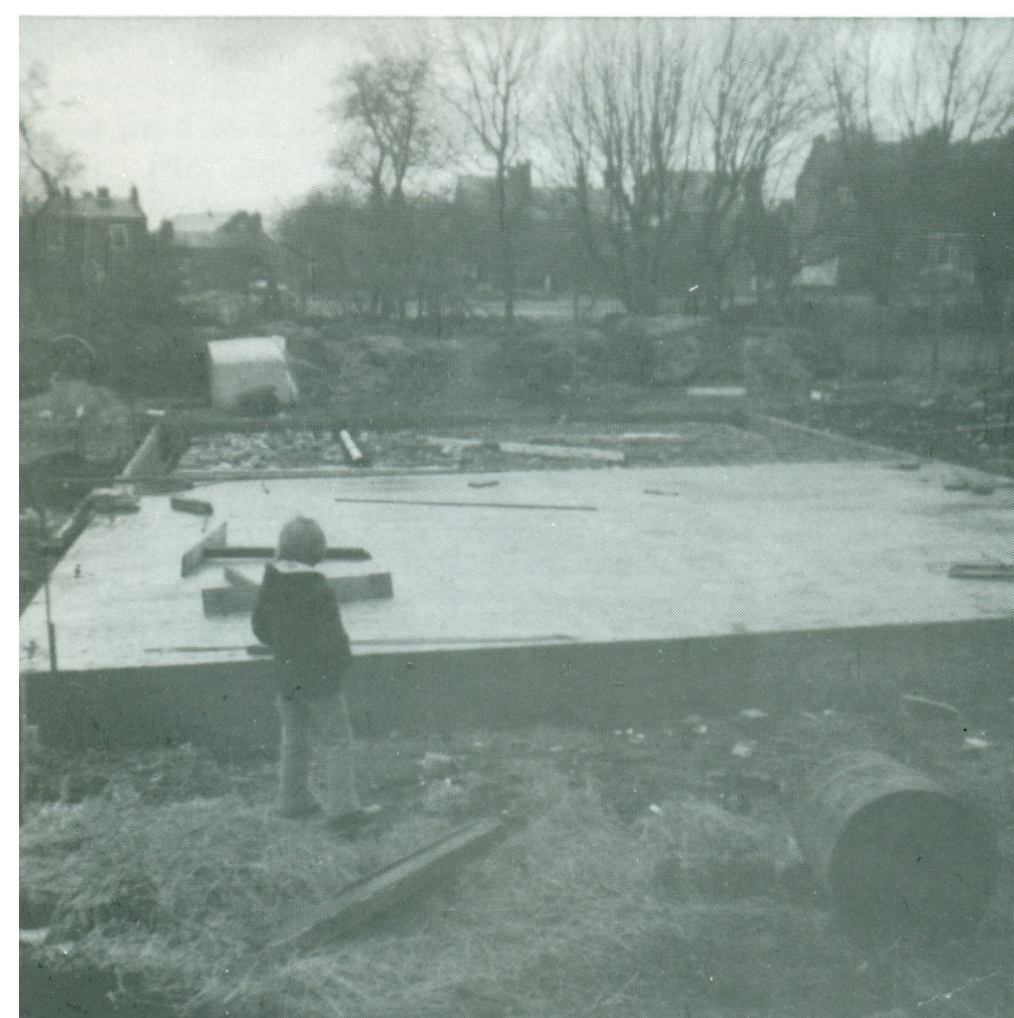
Contractors lay the foundations
