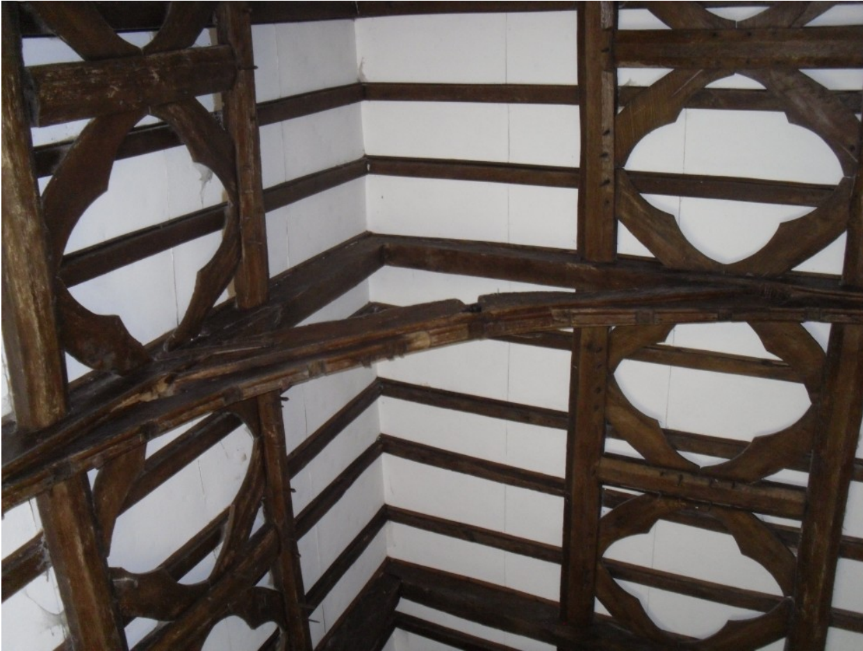
The roof at Stanton Long showing wind braces and quaterfoils.
