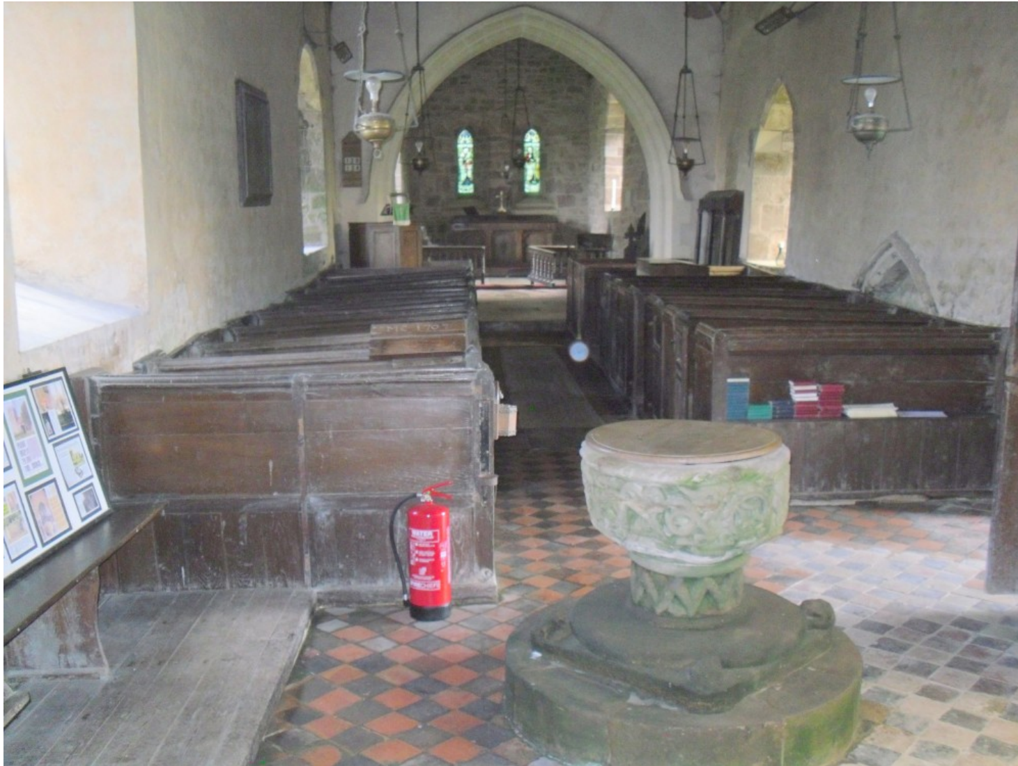
The inside of Holy Trinity, Holdgate. There is much restoration work needed.
