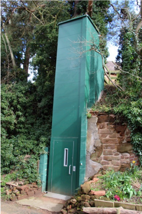
Access Lift for the congregation on service days at St Mary Magdalene, Quatford.
