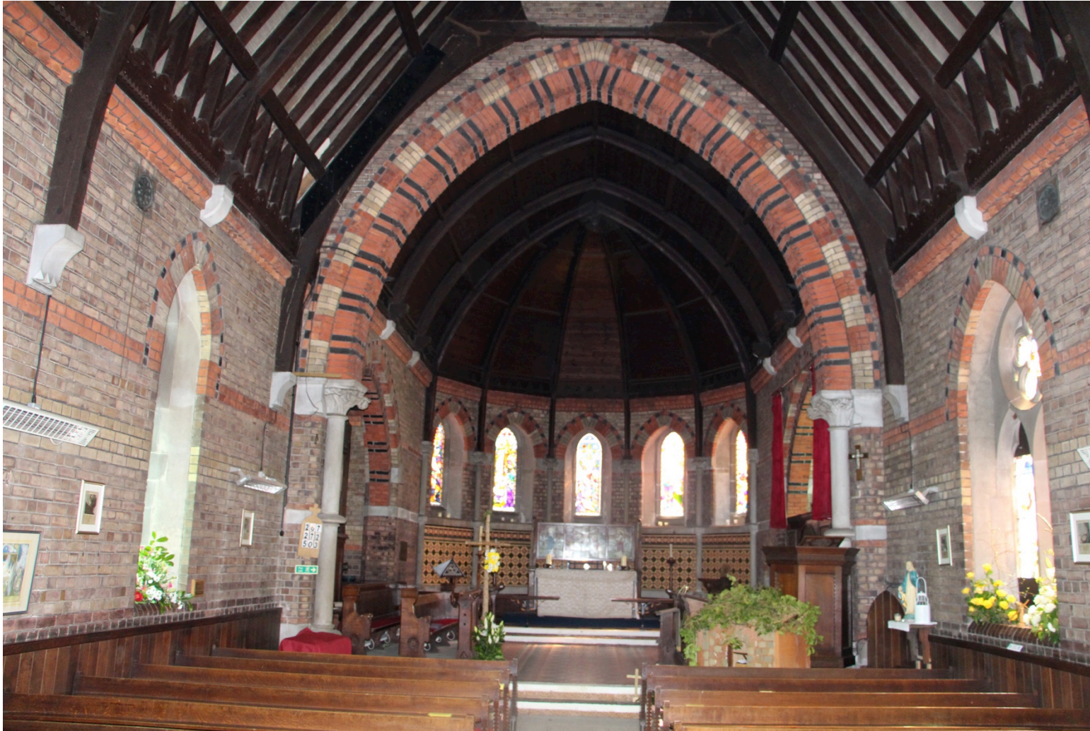
The nave and chancel at Jackfield. The chancel arch is made entirely from locally made bricks.
