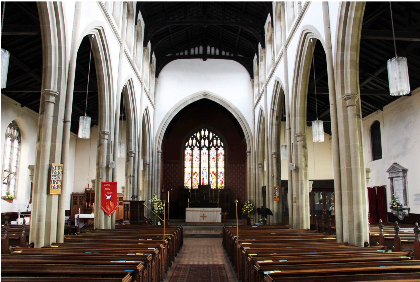
The central nave is 46 ft high. Stone arched columns divide the central nave from the north and south aisles. Galleries over the aisles were removed in 1980.
