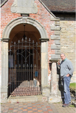
The brick south porch at St Giles, with pedestal structure at the entrance.
