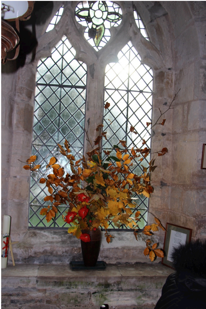
Tracery in the south window of the nave.
