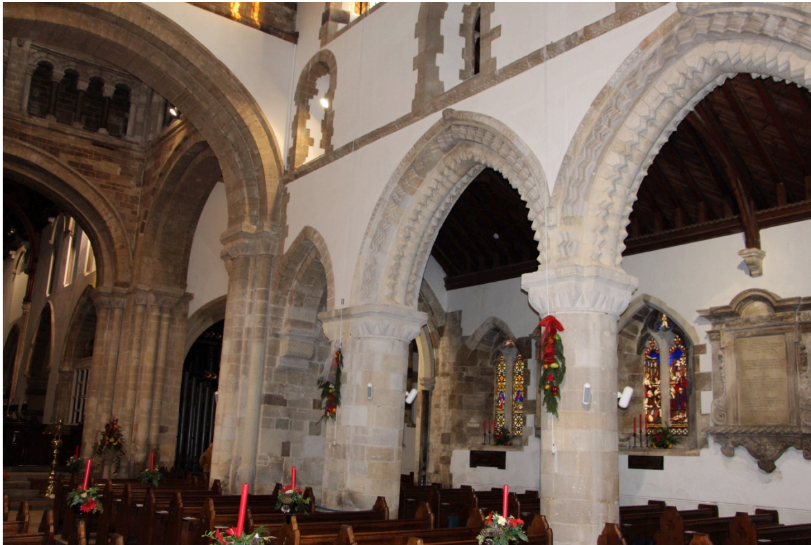
The arches in the nave at Wimborne Minster.
