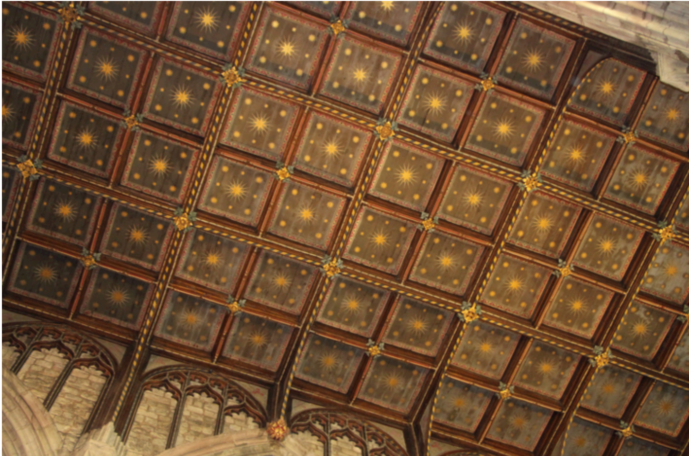
Ceiling tiles at Great Malvern Priory installed during the restoration of 1860.
