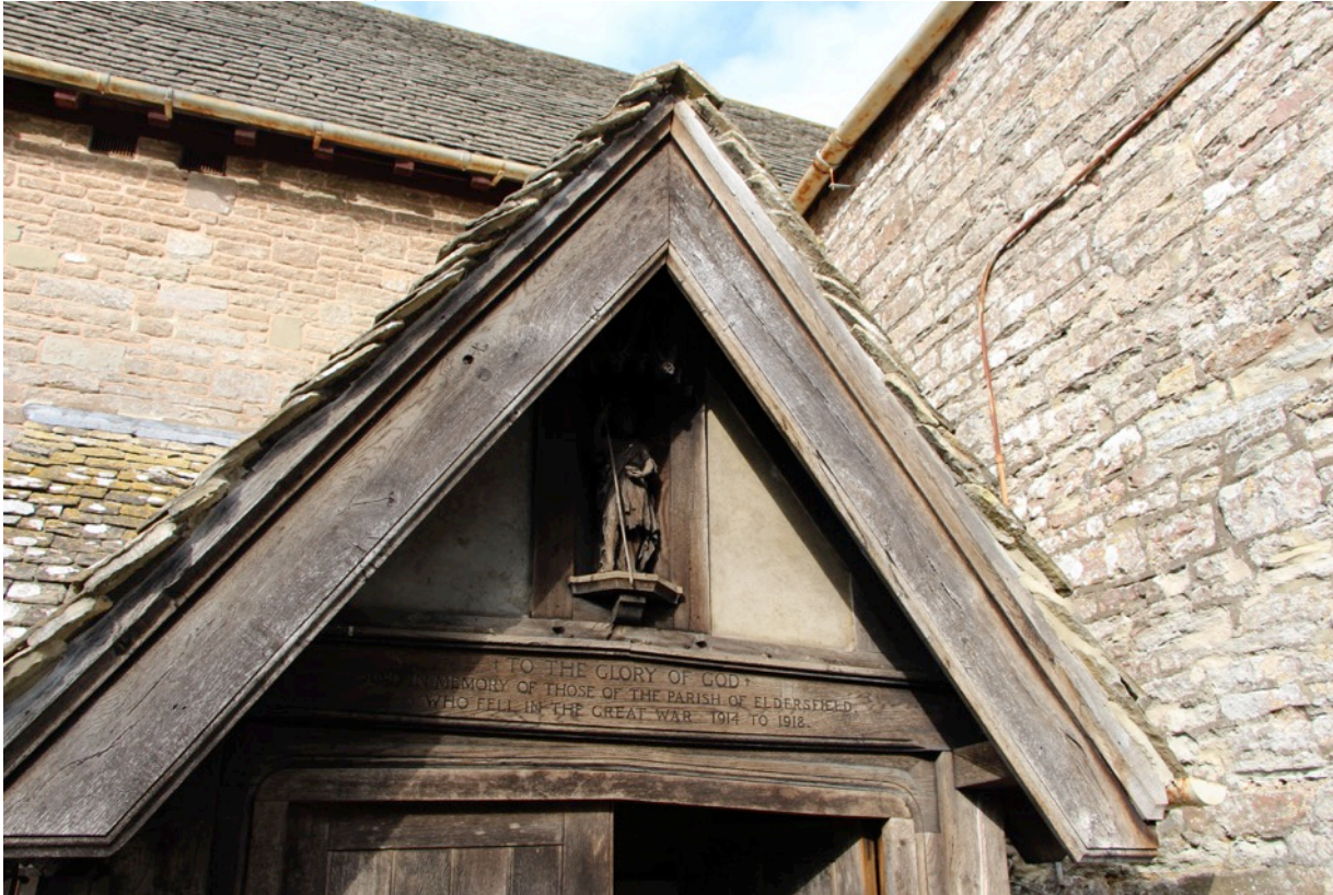
War memorial porch at St John the Baptist, Eldersfield, Diocese of Worcester.
