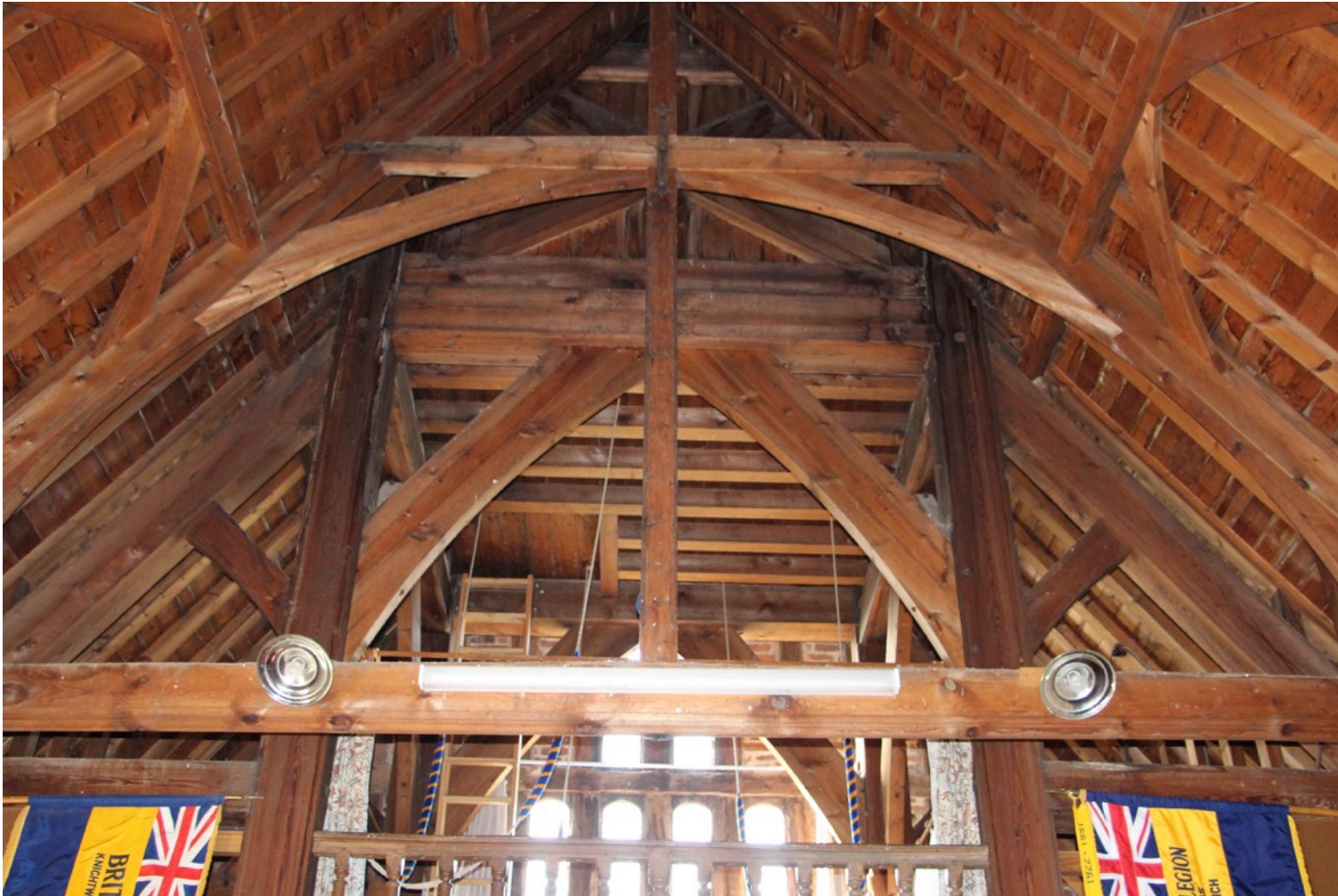
The extraordinary roofwork construction at St Mary Magdalene, Broadwas.
