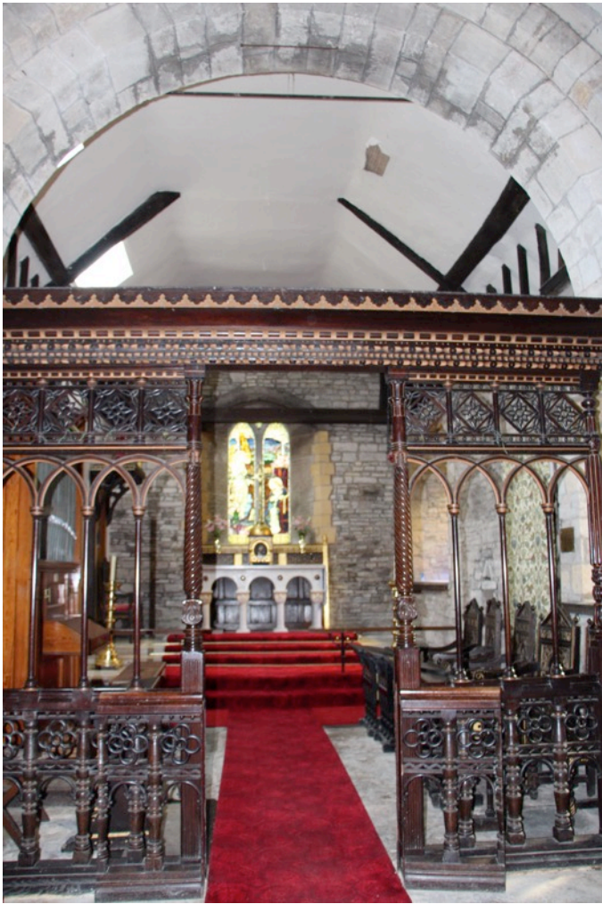
A very elaborate intricately carved rood screen divides the nave from the chancel at St Peter's, Rous Lench.
