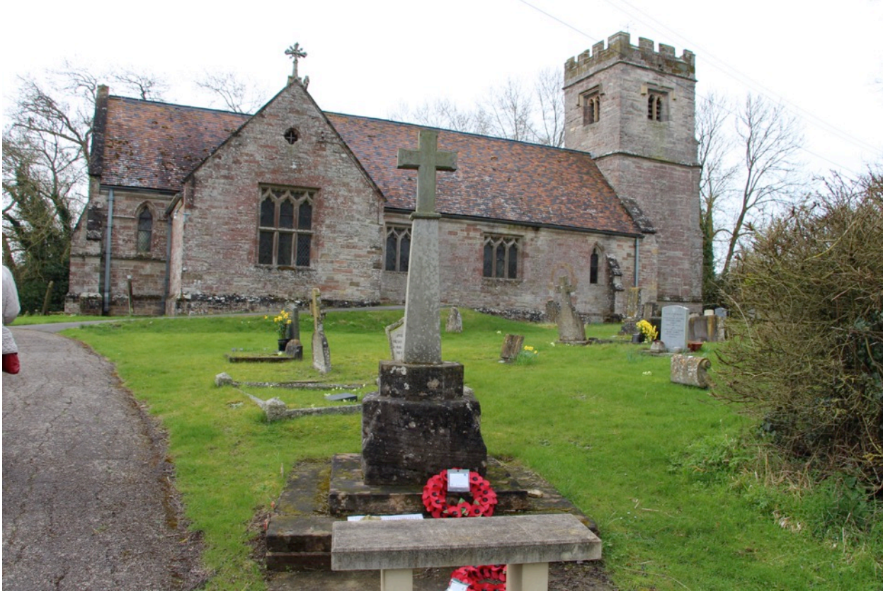
The exterior of St Peter's Church, Flyford Flavell.
