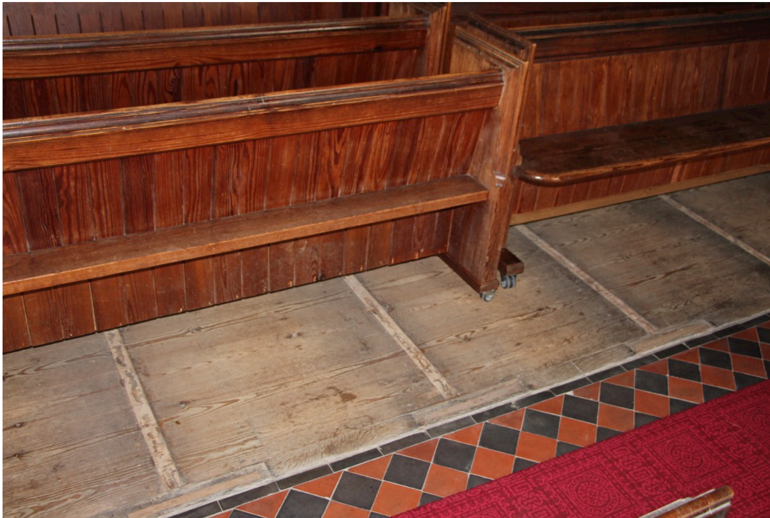
A novel solution to church reordering seen at St Peter's, Flyford Flavell: the pews have been retained but are now fitted with casters, enabling them to be moved out of the way easily.
