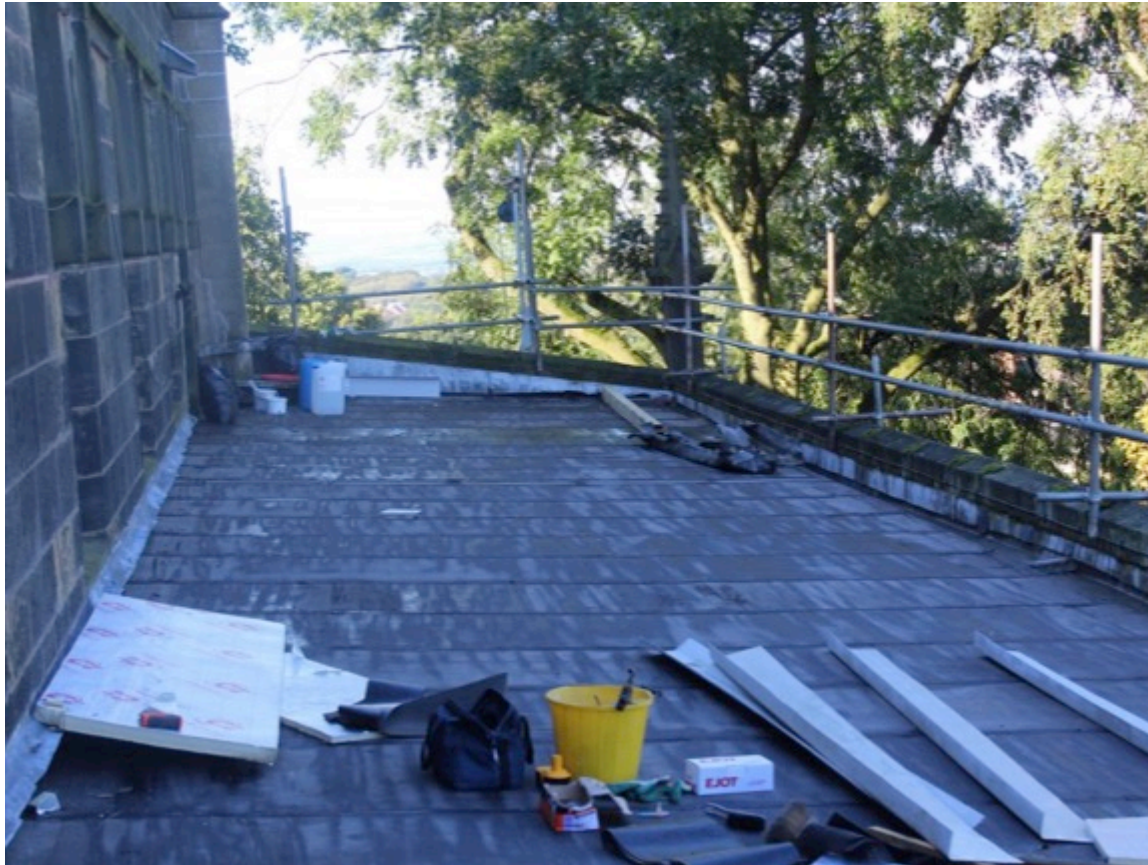
Roof repairs in progress, after lead stolen, 2016
