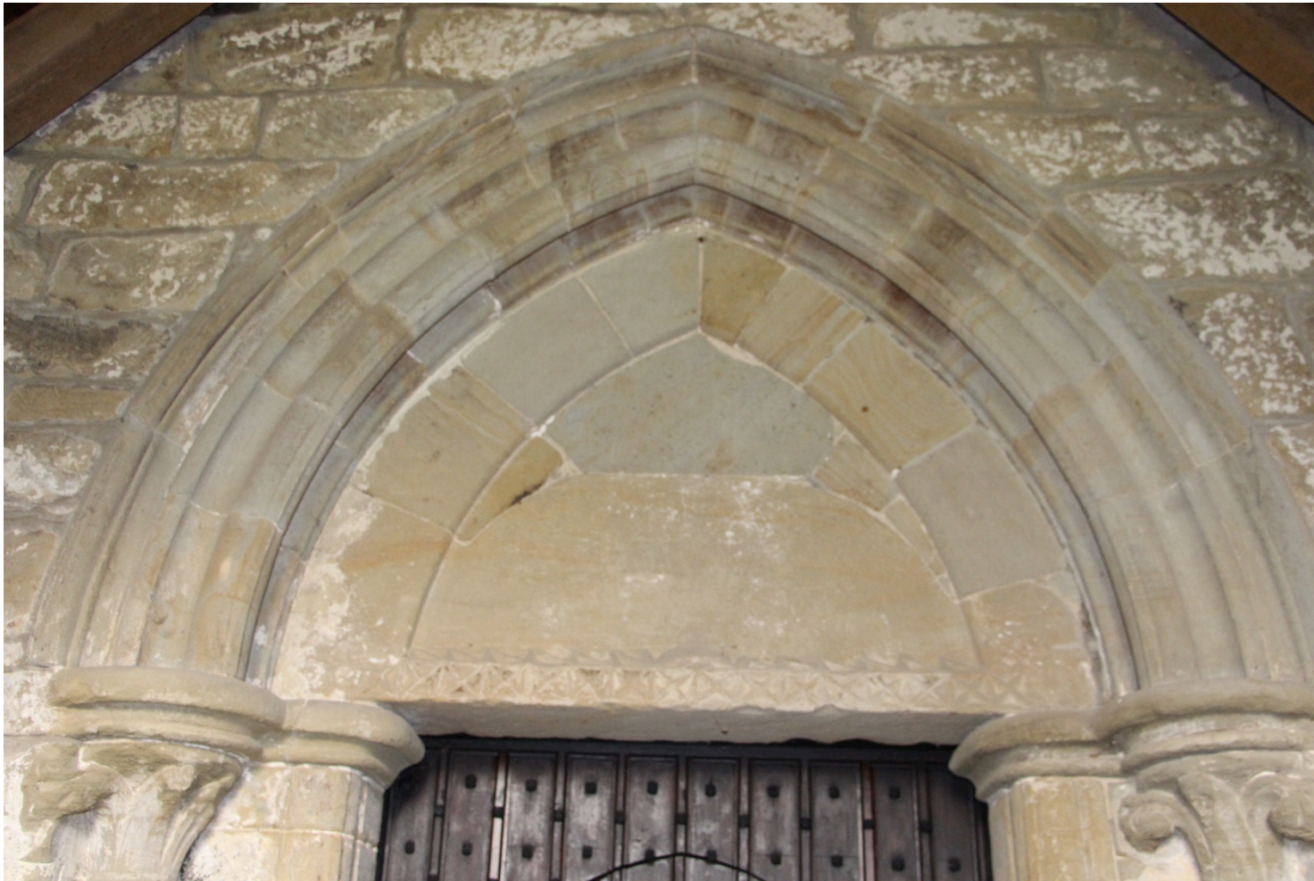
Above the south door is a tympanum with dogtooth moulding below – it dates from the 12 th century when the early Norman church was built , and is incorporated into the porch.
