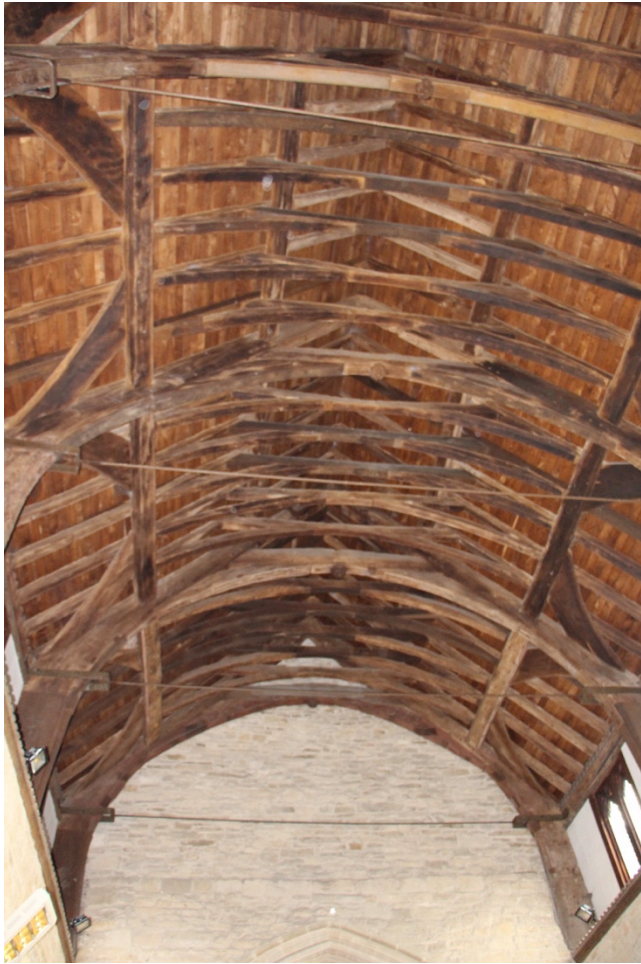
The tie-beamed roof to the nave; stone heads carved into the tops of columns at the rear of the nave.
