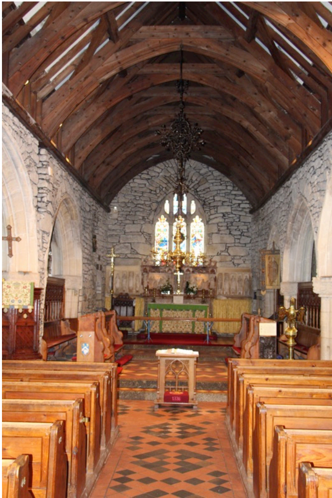
The nave at St Just in Penwith – the roofs of many Cornish churches resembles the structure of an inverted boat.
