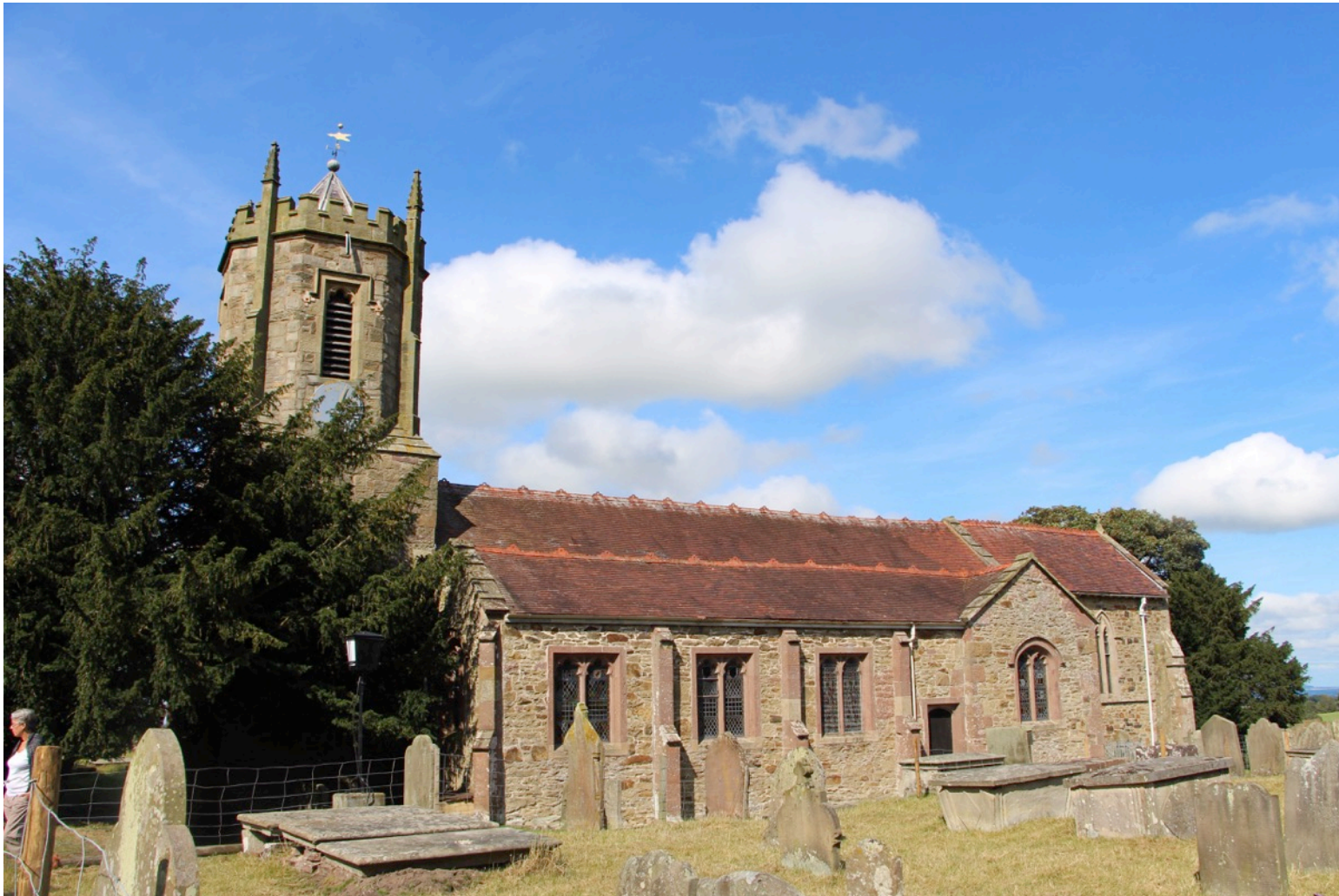
St Mary the Virgin, Dudleston. Much of the church is 19 th century – rebuilding and enlargements taking place in 1819 and 1877.
