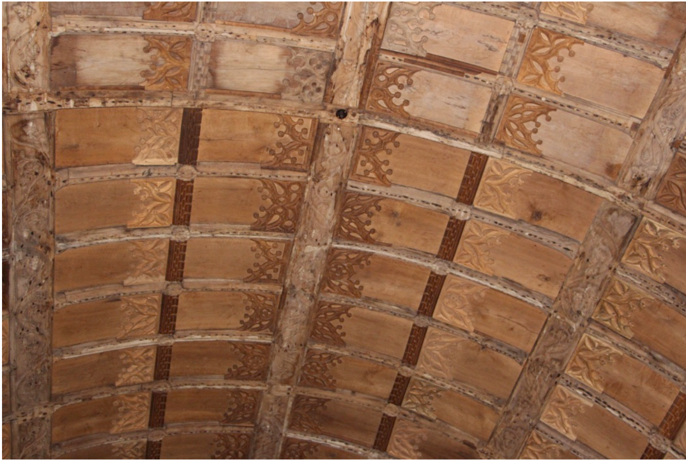
Another part of the roof at Selattyn.
