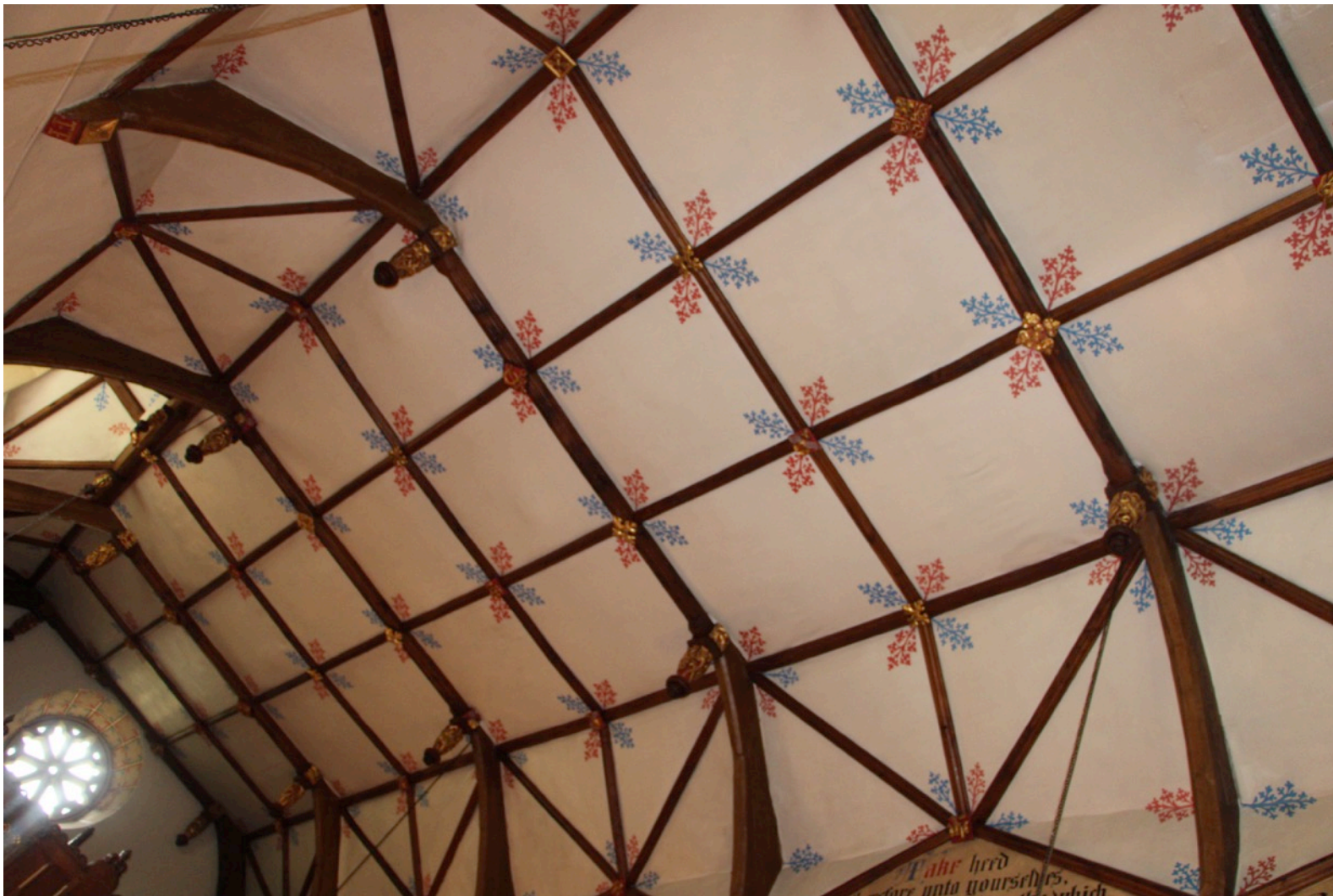
The ceiling, with sculptured ceiling bosses and decorative stenciling.
