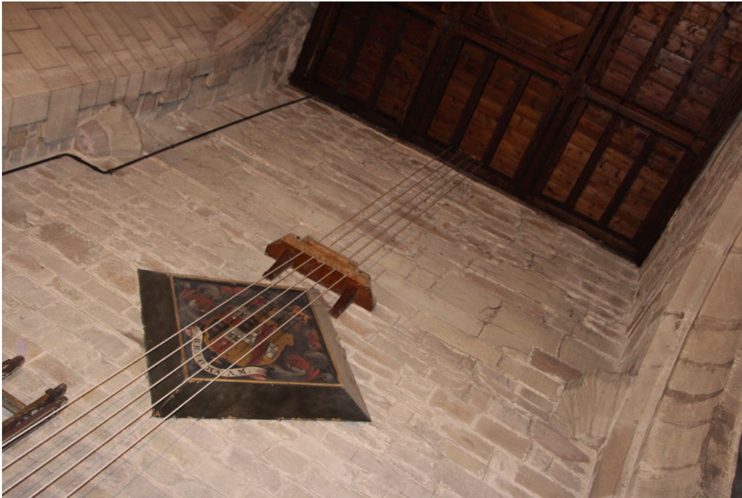
The bell tower, with hatchment. The wires are attached to a carillon - a stationary set of five chromatically tuned bells in the tower, played from a keyboard .
