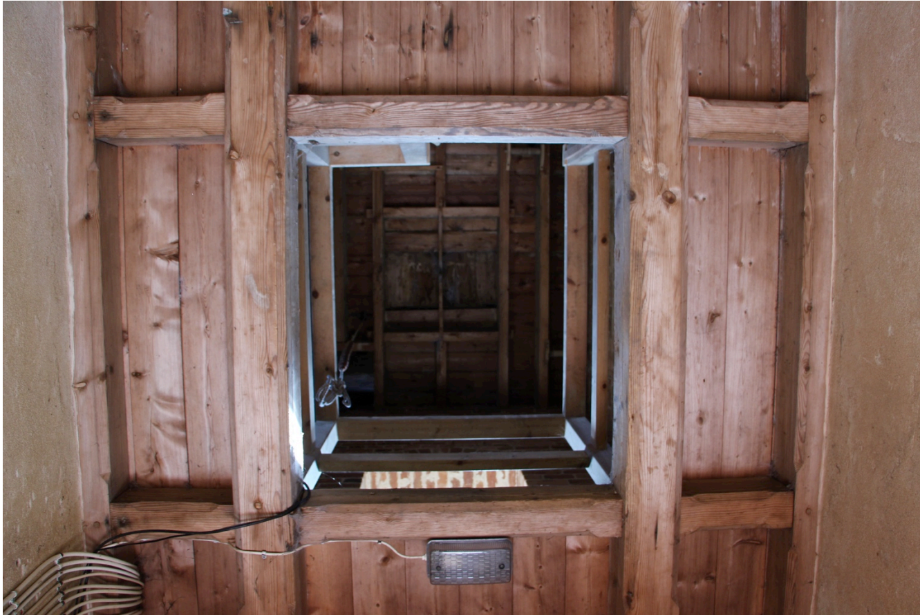
The tower and bell ringing gantry at Holy Cross Bobbington. Nowadays the bells are operated by an electronic carillon.
