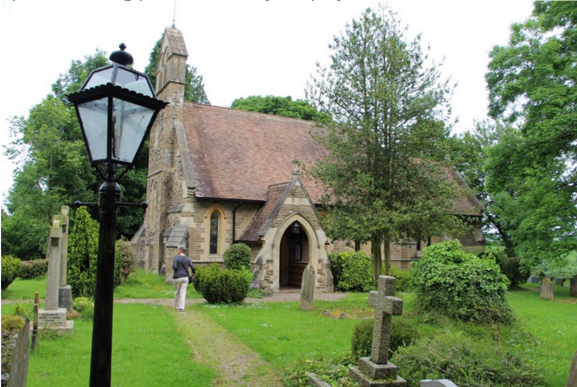
The new St Bartholomew's church, in nearby Harpley.
