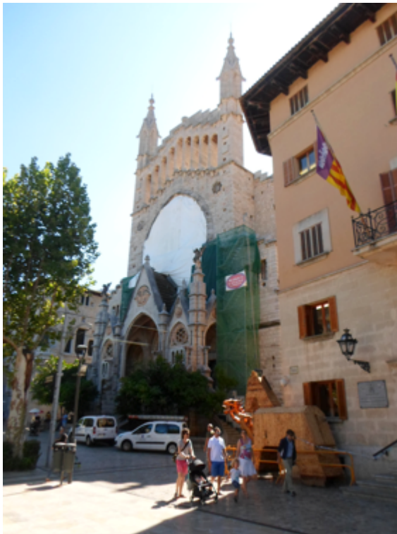
The church of St Bartholomew in the Placa Constitucio in Soller. Its oriel window was under repair.
