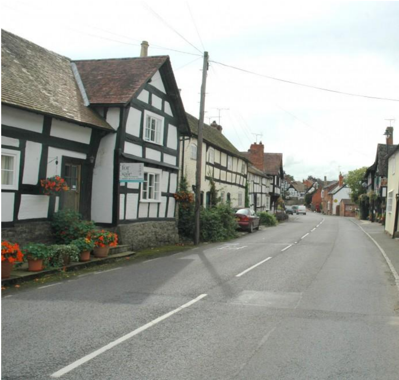
Pembridge High Street, wide view
