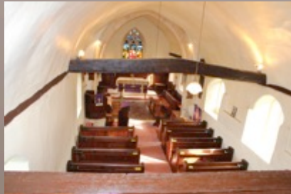
Tie Beam Roof, Defford
