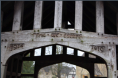
Lych gate memorial, St John the Baptist, Beckford
