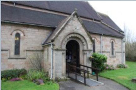
Exterior: The Bridge, Headless Cross
