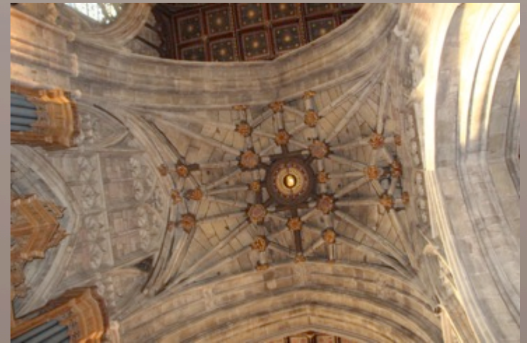
Vaulted ceiling, Great Malvern Priory
